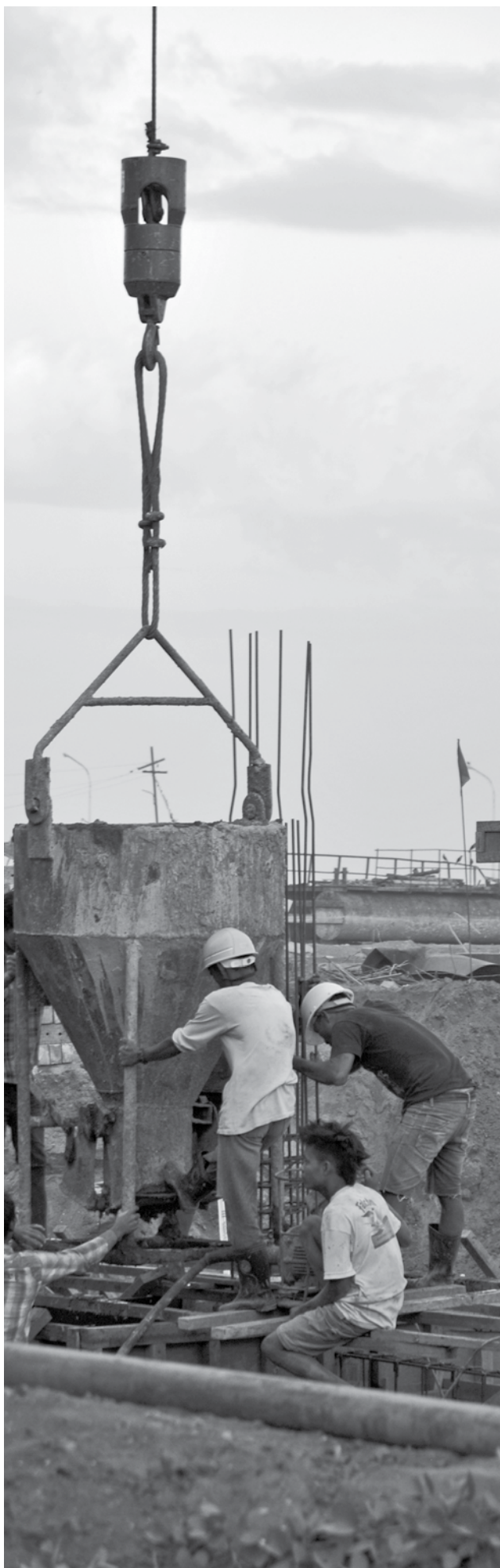
The Kaladan Project, working on expansion of Sittwe port (TK)
